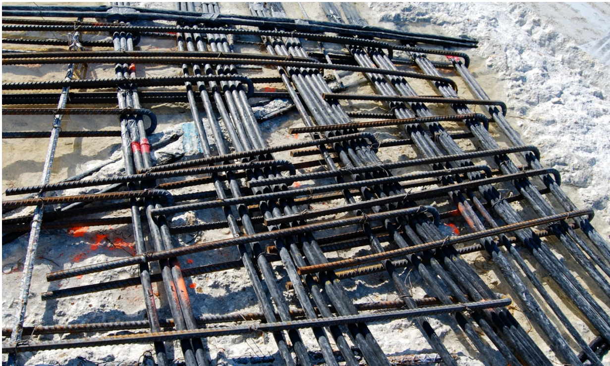
Photo: Supplemental hairpin reinforcement added at banded tendon lateral sweep repair.
