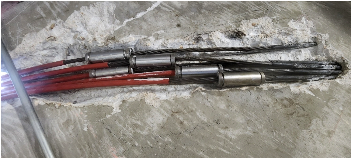
Photo: Installation of these splice couplers within the tendon sweep places an eccentric load on the hardware.
